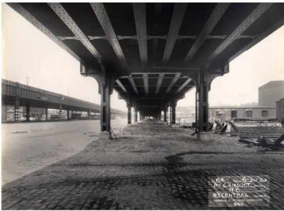
High Line during construction. Underside view
