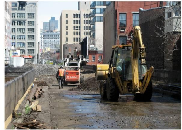
Diggers on High Line working on site preparation
