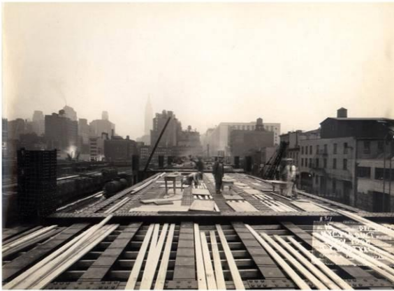
High Line during construction. Topside view
